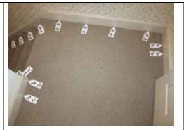
8- Align the long edge of a Landing marker along any bulkhead or possible upper obstructions to a lift passenger's head.
