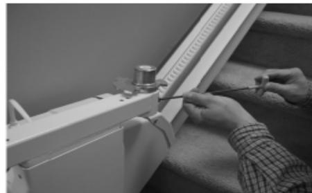
Position the seat assembly on the Seat Swivel Post ensuring that the swivel lever is depressed so that the seat is fully engaged with the swivel post. Check the swivel lever to test the locking mechanism.
