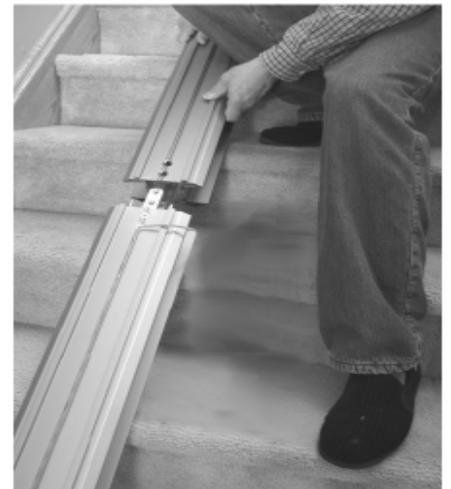
Install the 2 joint fasteners and firmly tighten with 5/16" Allen wrench (bottom side).
