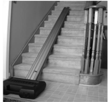
Position the two ends of the track close together. Locate and connect the plug on the ends of the two charger harnesses inside the two track pieces.
